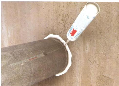
Acrylic, intumescent based material with excellent adhesive properties for fire resistant sealing of joints and service penetrations for up to 4 hours FRL when tested to AS 1530: Part 4, AS 4072: Part 1 and BS 476: Part 20.
